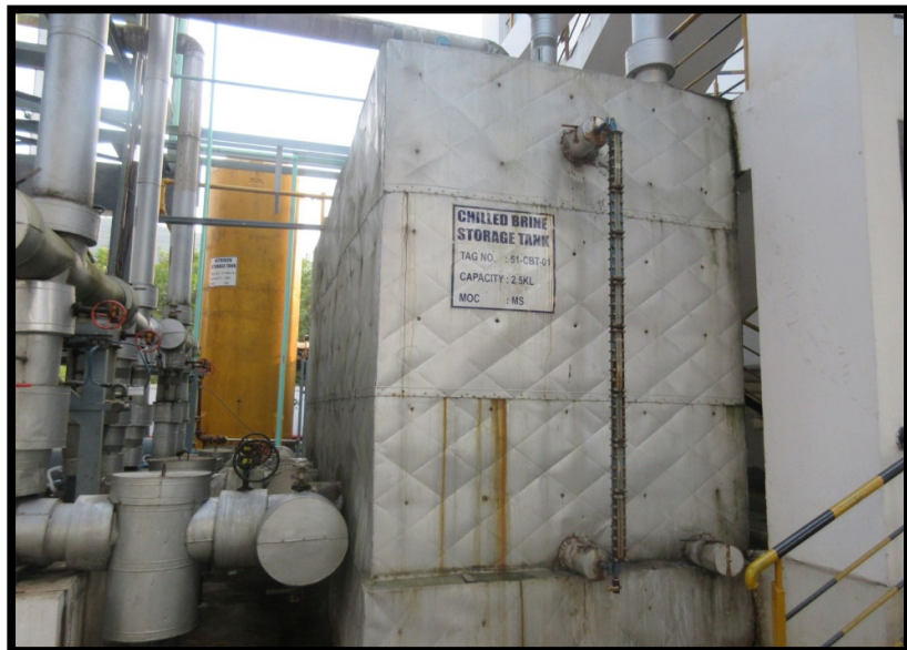
CHILLING BRINE STORAGE TANK
