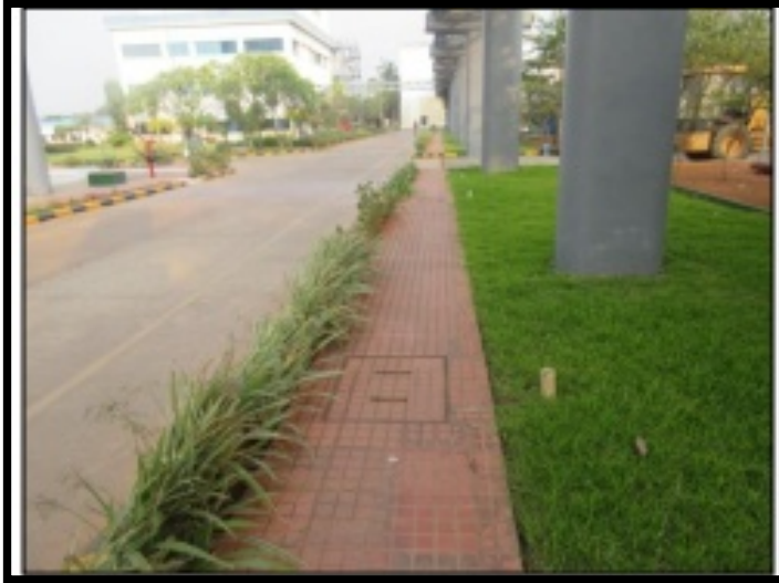
STORM WATER DRAIN
