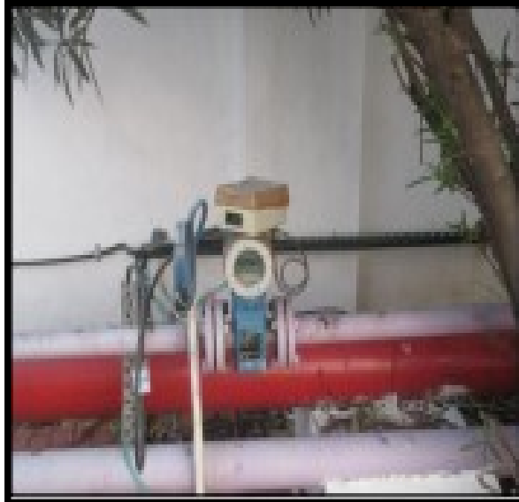
DIGITAL FLOW METERS AT FRESH WATER FACILITY
