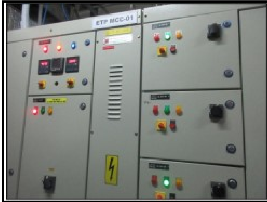
ENERGY METERS FOR ETP & APCE
