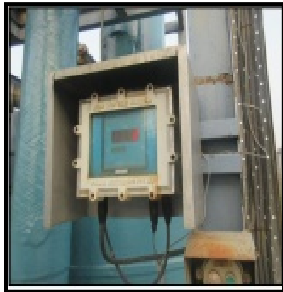
ONLINE pH METER CONNECTED TO MULTI STAGE SCRUBBER
