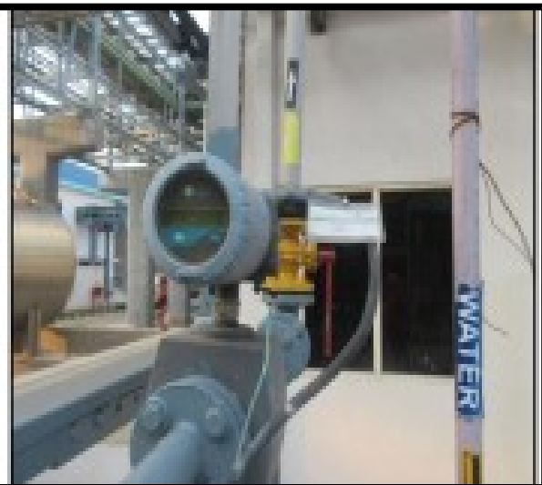
DIGITAL FLOW METERS AT PROCESS AREA FOR LTDS & HTDS
