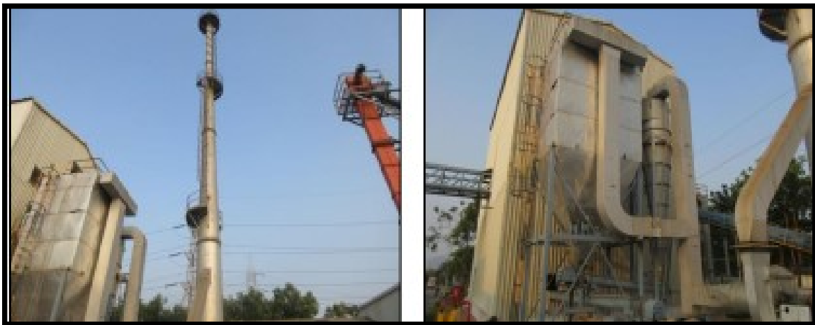
BOILER STACK, AIR POLLUTION CONTROL DEVICES (CYCLONE SEPERATOR & BAG FILTER)
