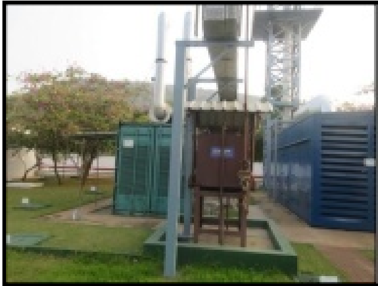
DIESEL GENERATOR WITH ACOUSTIC ENCLOSURES
