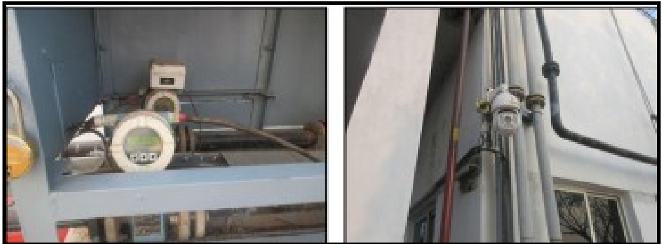
EFFLUENT FLOW METER & WEB CAMERA FACILITY
